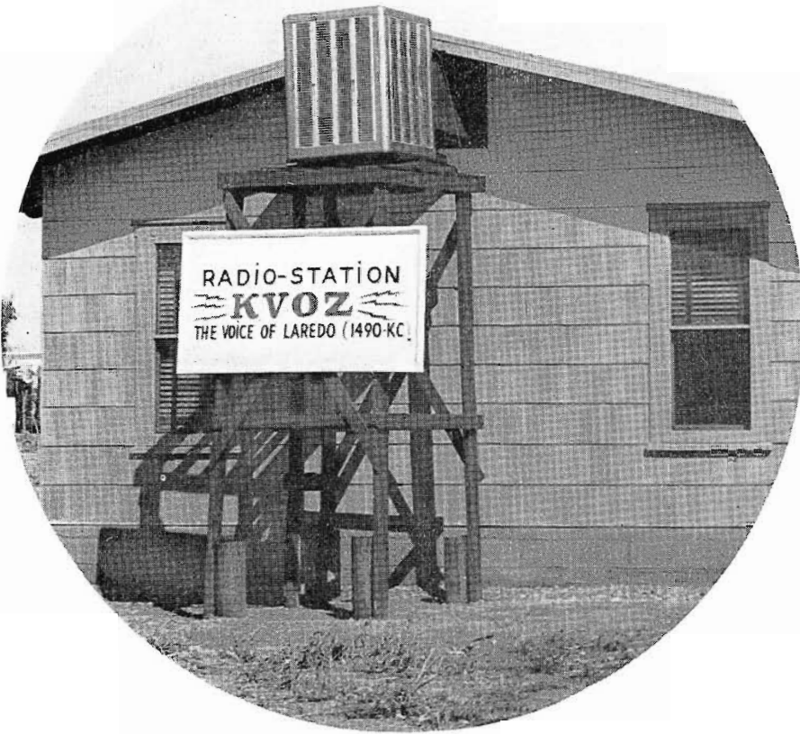
FIG. 1. Air-cooling is a "must" in Laredo where temperatures reach a maximum for the United States.
