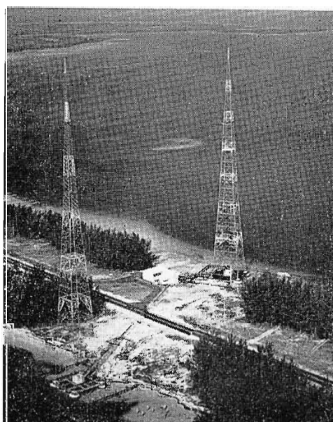
FIG. 9. Aerial view showing complete WSUN tower-transmitter layout. Two 500-foot towers straddle over-water highway connecting St. Petersburg and Tampa.
