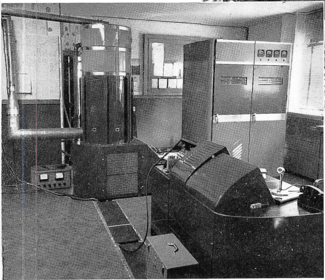
FIG. 6. Shown at right in this photo (not visible in Fig. 5) are the visual power and control cabinets and the operator's console. The aural power and control cabinets (not visible) are located at the opposite end, just behind the console.
