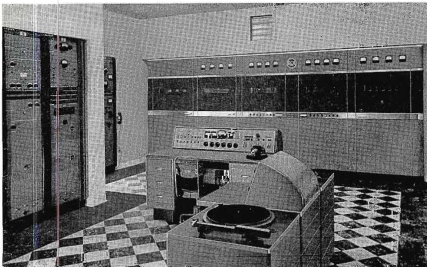
FIG. 4. Transmitter control room showing RCA 5-KW BTA-5F. Phasing equipment in left cubicle. Transmitter control desk, turntables and special audio console in center foreground.
