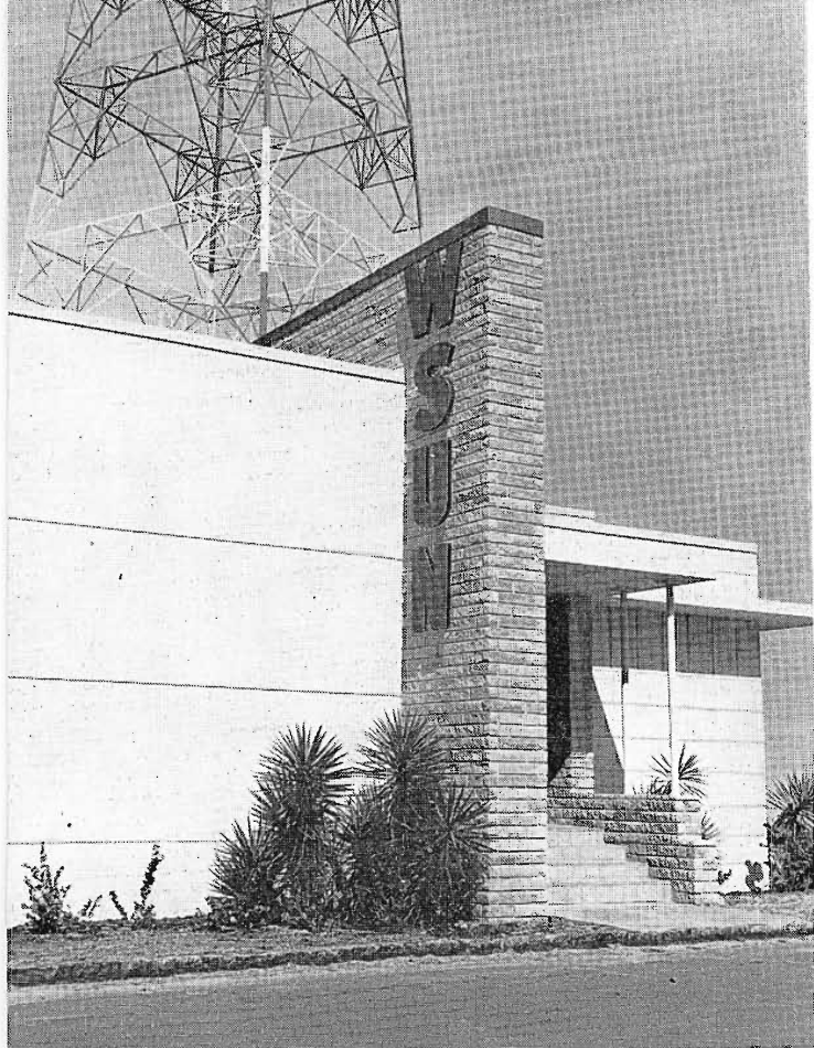
FIG. 1. Entrance to the WSUN transmitter building, with the northwest tower rising in the background.
